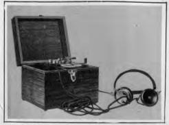
RADIOLA JR. is a complete Radio receiving outfit. Its range varies from ten to twenty miles. The only adjustments necessary include the occasional finding of a "sensitive spot" on the crystal detector and the simple turning of a tuning control arm to cover the wave length range of 190-500 meters. Built in a very substantial and attractive wood cabinet, the receiver has a compartment for storing the telephone receivers when the set is not in use.
