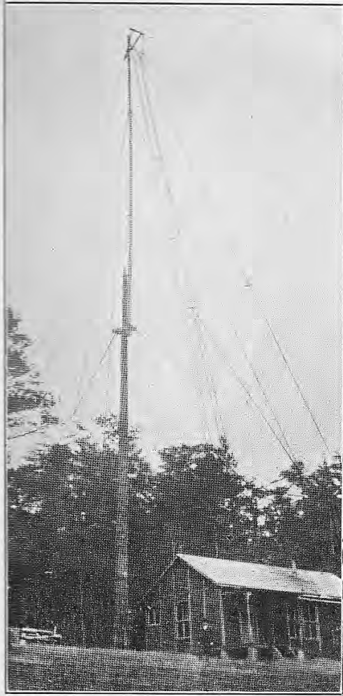
The Above is a Government Station from which the Pacific Received Toll for Three Years
