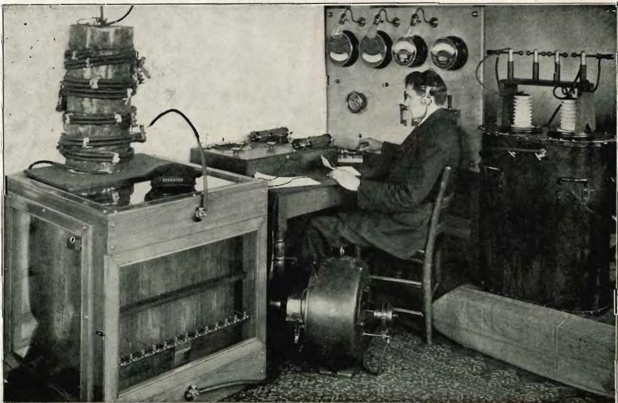
INTERIOR VIEW CLARK WIRELESS TELEGRAPH STATION, BUFFALO, N. Y.
