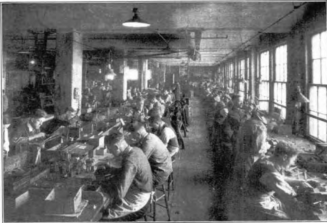
Light-Assembly Room of Main Plant of WIRELESS SPECIALTY APPARATUS COMPANY
