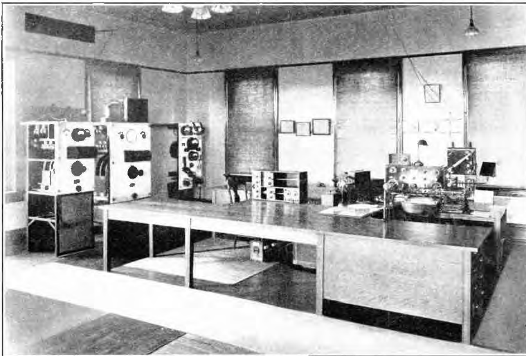
Operating Room of the New Orleans Station of the Tropical Radio Telegraph Company, equipped with WIRELESS SPECIALTY APPARATUS COMPANY'S Auxiliary Transmitter and Receiver
