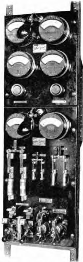
LOW-TENSION CONTROL PANEL
