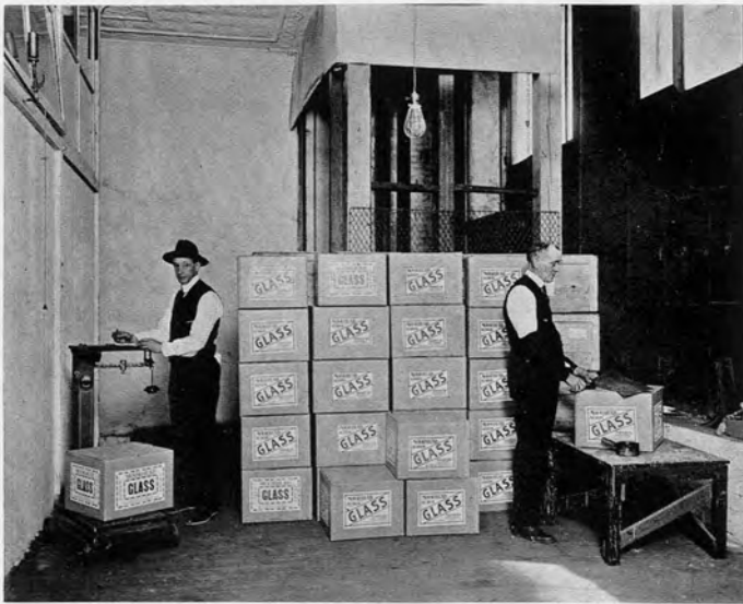
Moorhead Laboratories Section of Shipping Department.
