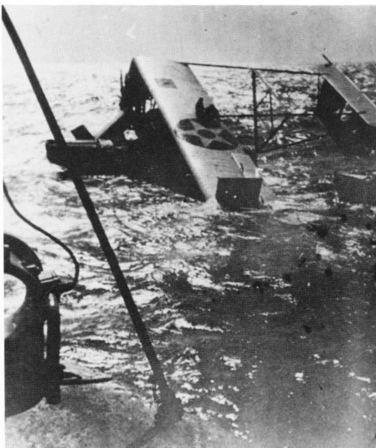
NC-5, damaged under tow, was sunk by gunfire in 1921.
