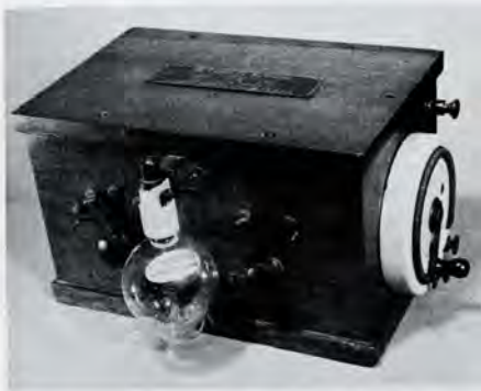
Figure 9 - Improved Type RJ4 Detector
